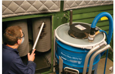
A clogged filtering system for a buffing booth is quickly cleaned and put back into service using the Heavy Duty HEPA Vac.
